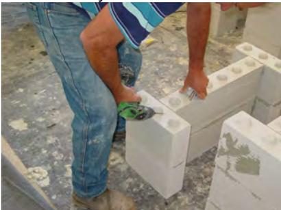
Fixing connectors on one end
