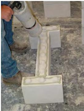
Spreading mortar for the second layer of blocks
