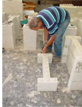
Screw driven from outer block to inner block
