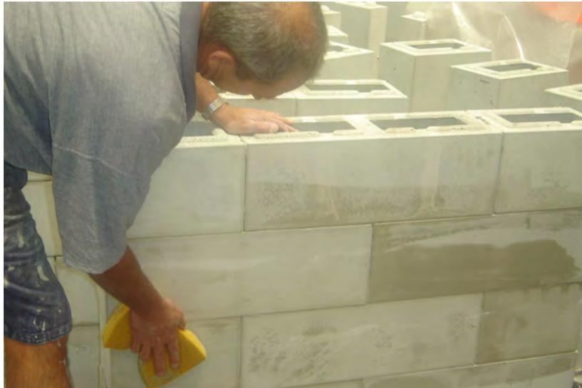
**Figure 6.** Finishing the surface of the wall
