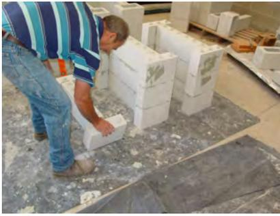
Gluing the first layer of blocks
