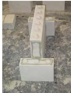
Mortar on the header face and bed face
